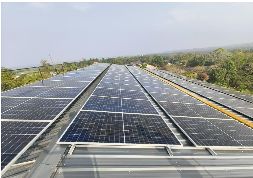
Fig. 2. Full perspective of the KCAEFT 100 kW rooftop installation showing both Left Grid and Right Grid alignment, metal sheet roof substrate, aluminium racking structure, and surrounding tropical landscape of Malappuram District. (Source: Field photograph, KCAEFT campus, December 2024.)
