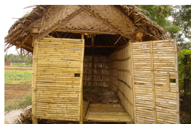
Fig.3. Low cost, bottom ventilated bamboo structure
