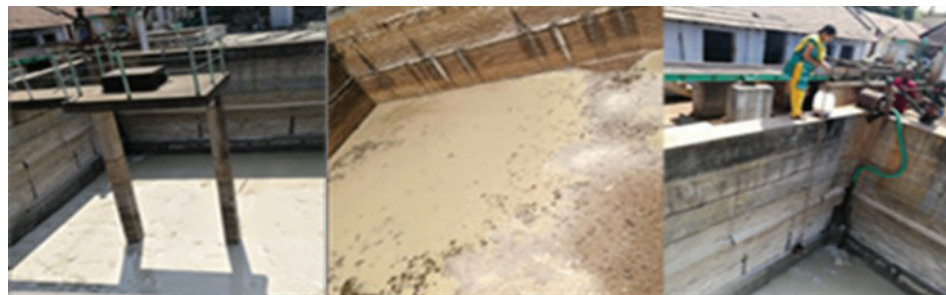
Wastewater storage tank and sample collection
